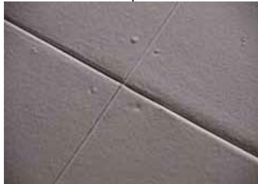
Photos 9 and 10: Examples where fasteners are fixed into the LDB sheeting and the edges are bevelled or slanted.
