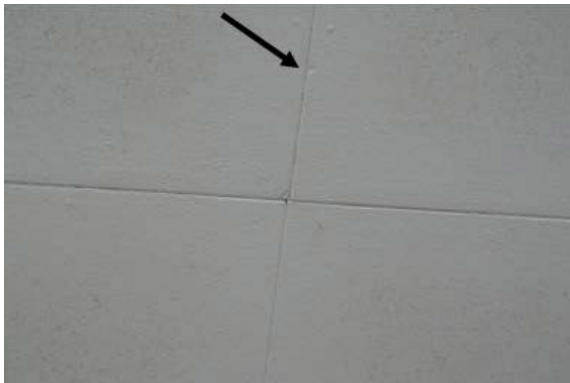
Photo 7: Recessed fastener heads in LDB.
